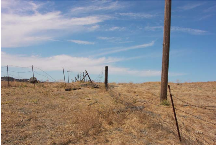
Figure 11 Damaged Fence Allowing Livestock Access
